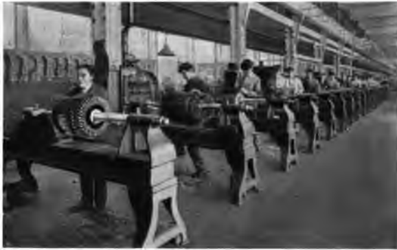
Winding Street Railway Motor Armatures, Section A
